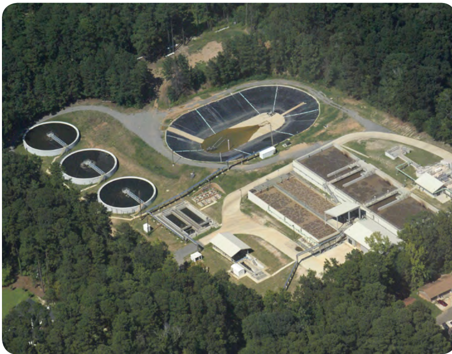
Image of the new state-of-the-art North Wastewater Treatment Plant.
